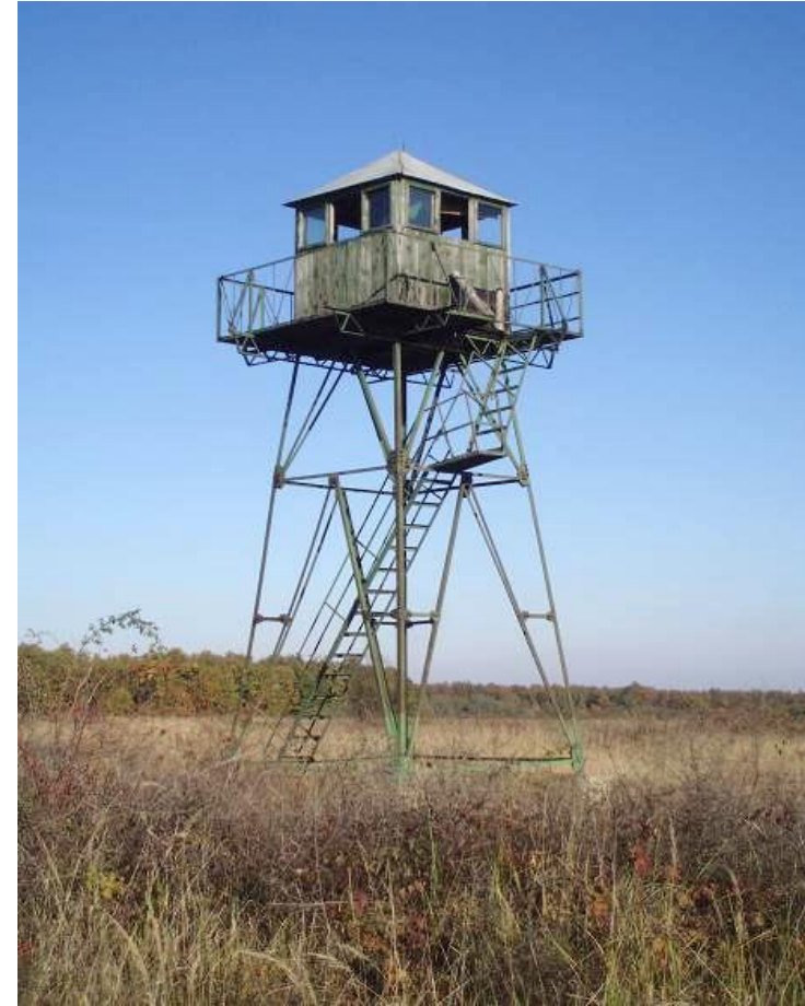
Bulgaria: Watch tower near Halovo
